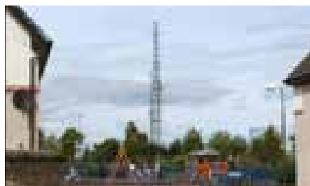
Photograph: West Granton Road, Edinburgh: a mast overshadowing a playground and housing. This breaks biological safety limits.
